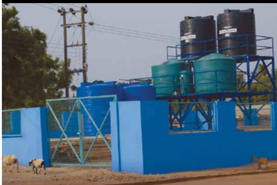
Safe Water Network's modular slow sand filtration system, Aveme, Volta Region, Ghana
